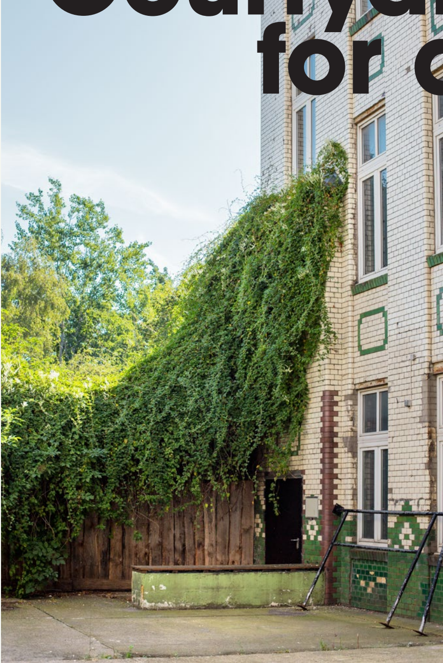
Photo: The PettCo's existing building prior to refurbishment
